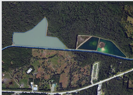
Figure 1: Aerial image of Beaufort-Jasper source water system including the treated reservoir.
